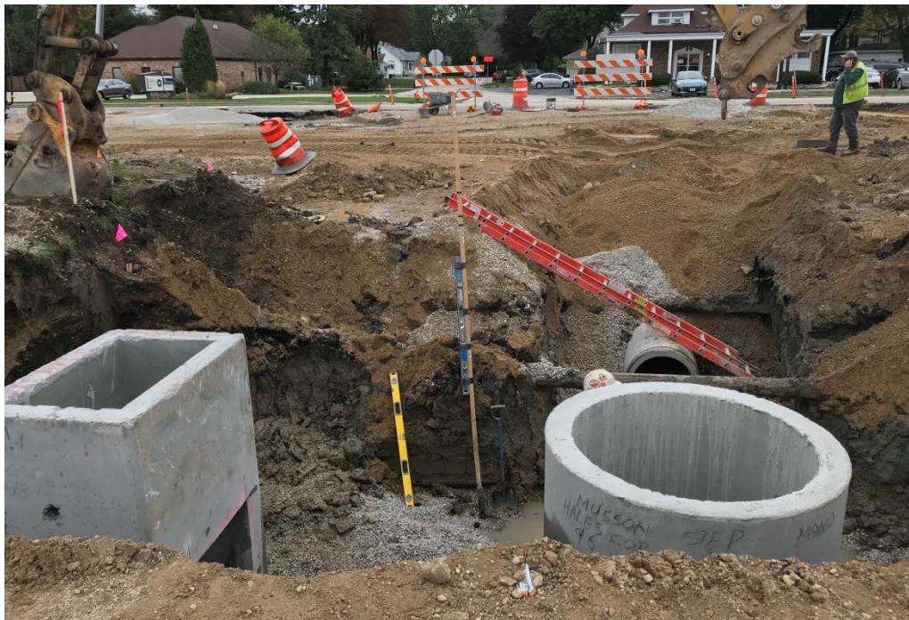
Installation of storm sewer inlets and lateral connection pipes along Hwy 100 south of Grange Ave.
