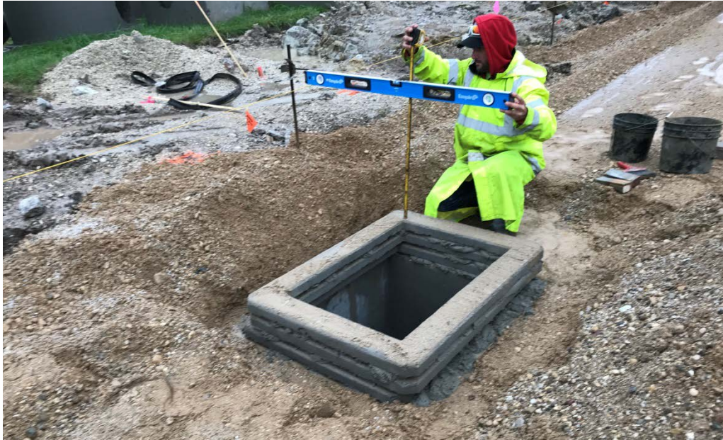
Adjusting storm sewer inlet elevation in preparation for curb & gutter.
