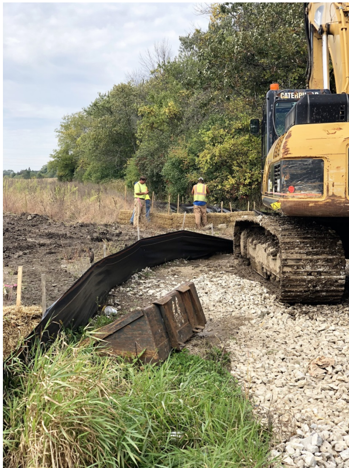
Installation of erosion control devices at the project fill site.
