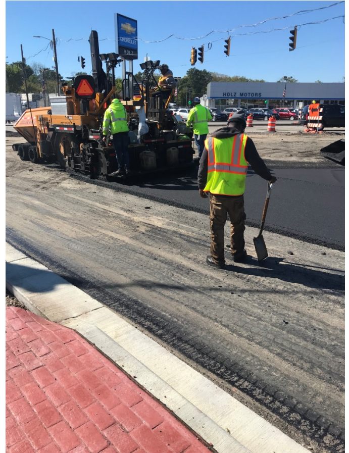
Placement of the surface layer of asphaltic pavement on the east legs of Janesville Rd. & Forest Home Ave.
