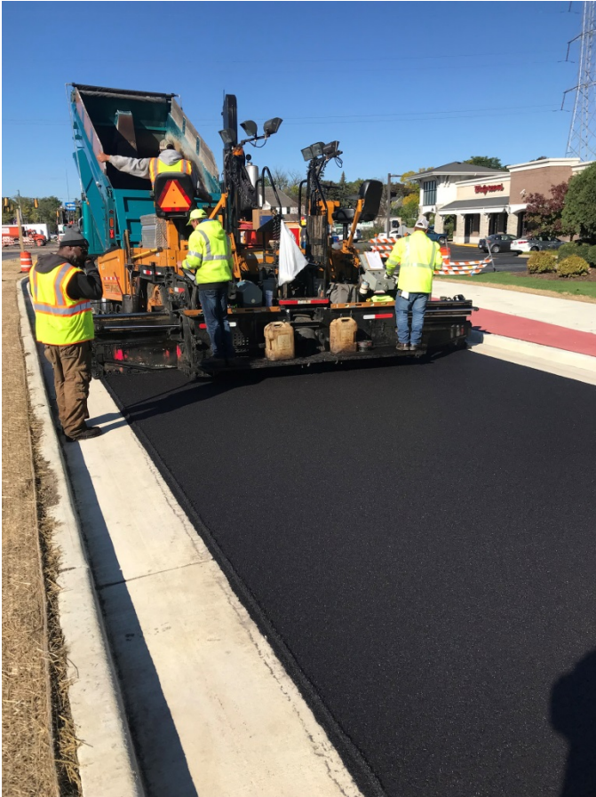
Placement of the surface layer of asphaltic pavement on the east legs of Janesville Rd. & Forest Home Ave.
