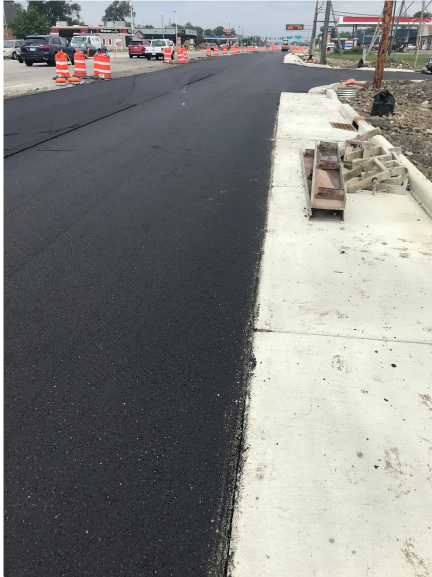
Placement of asphalt pavement along Hwy 100 between Edgerton Ave. and Copeland Ave.
