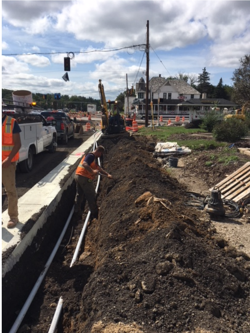
Installation of electrical conduit behind the curbline along the east leg of Janesville Rd.
