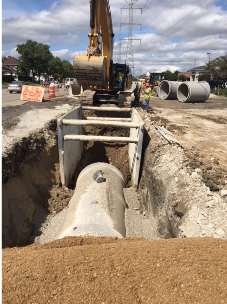
Installation of storm sewer trunkline north of Janesville Rd along Hwy 100.
