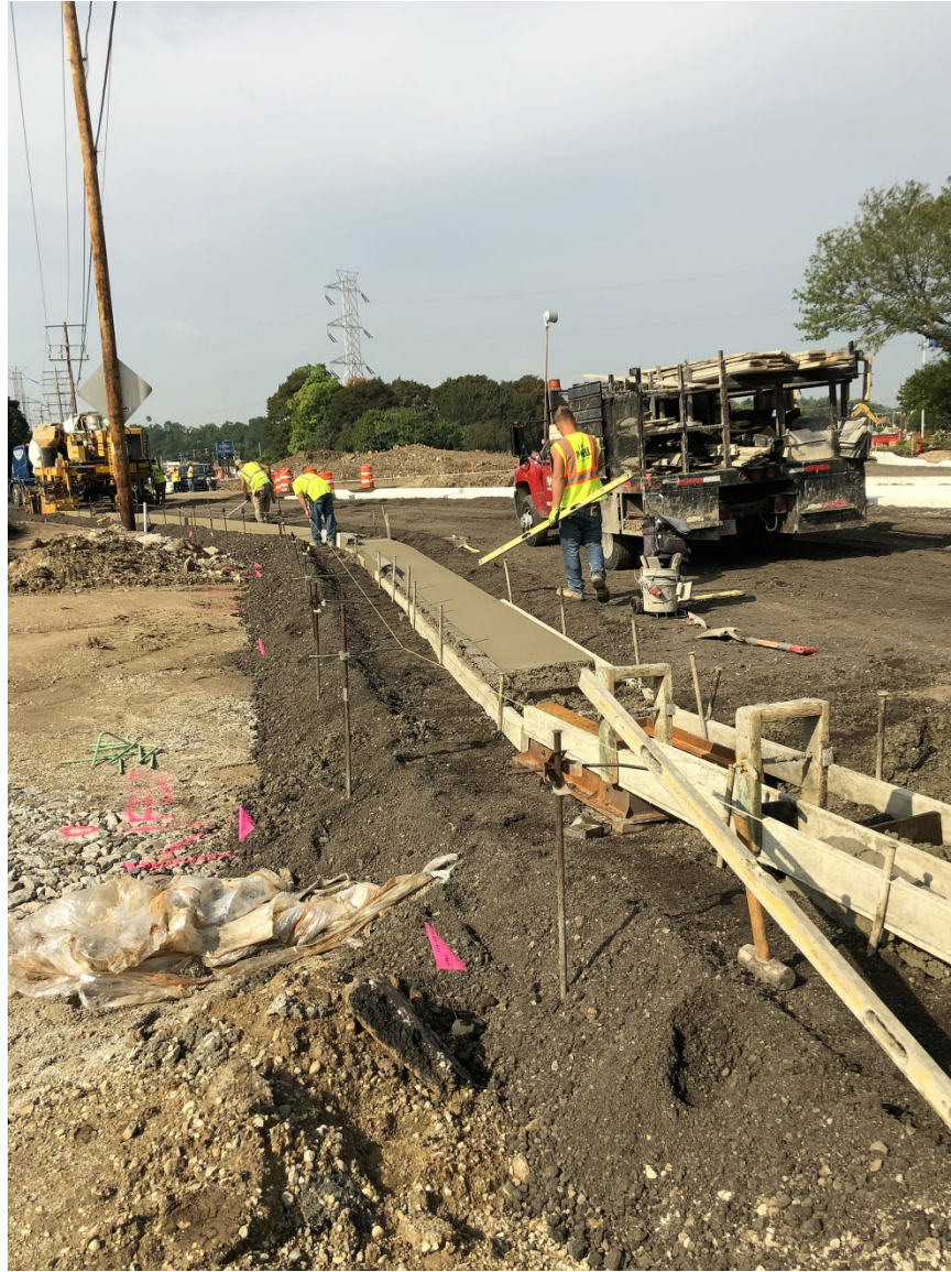
Placement of curb & gutter along the east leg of Forest Home Ave.
