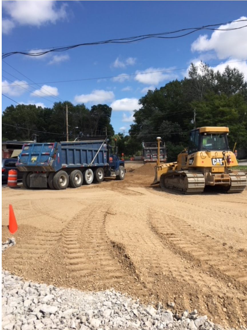
Placement of base aggregates on the south half of the east leg of Edgerton Ave.
