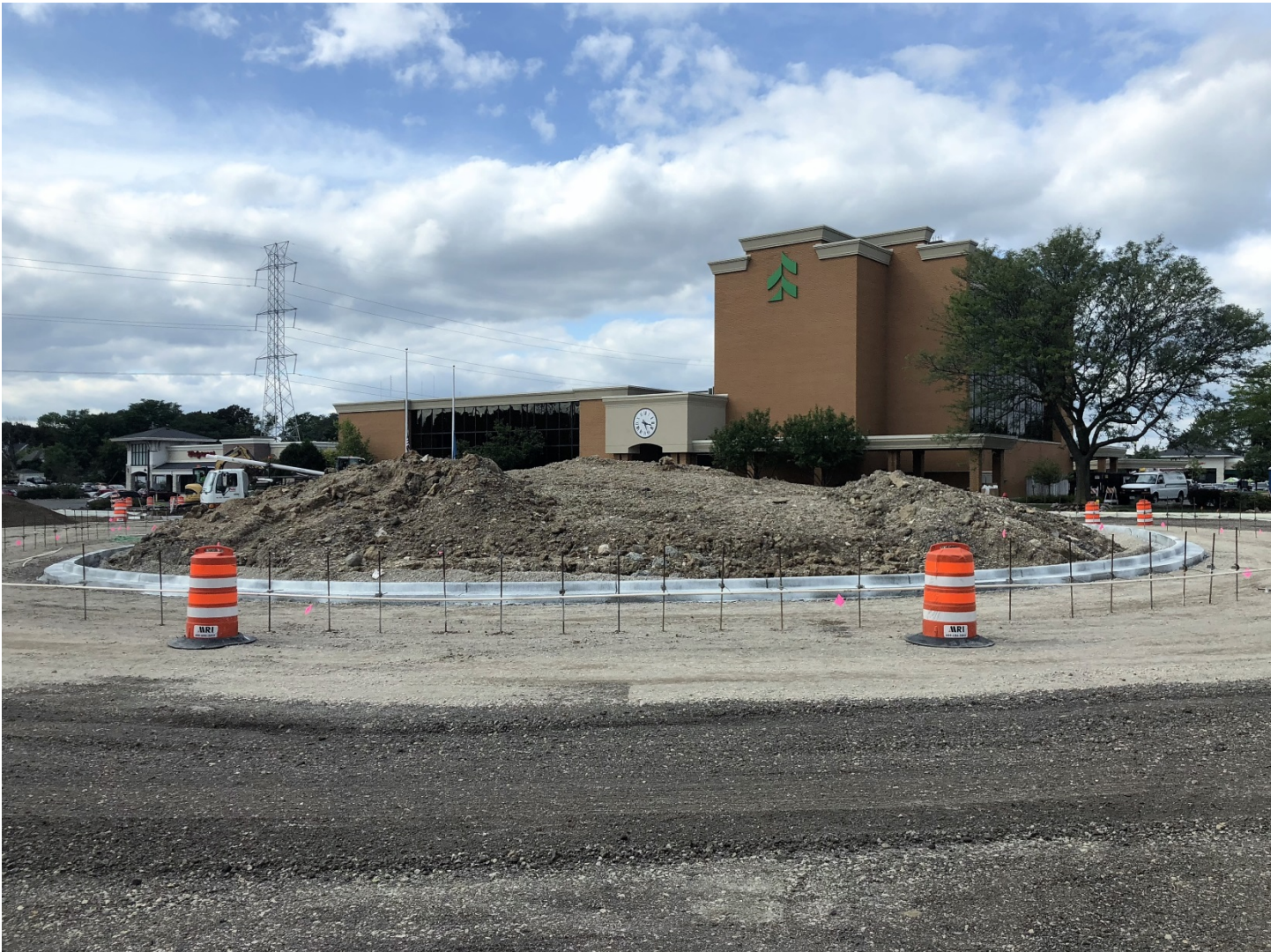
Concrete curb & gutter for center of Round-About at Janesville Rd-Forest Home Ave intersection.
